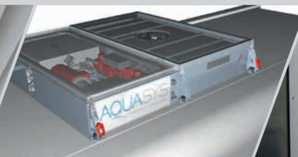
Water supply unit installation on the rooftop
